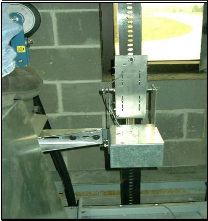
Figure 1.3: Typical Mounting of Selector
