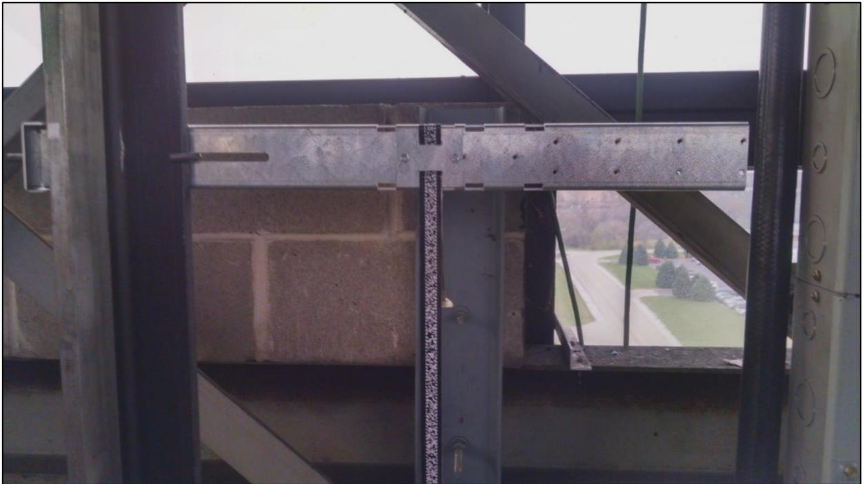
**Figure 2-1: Encoded Tape Mounting – Top Bracket**
