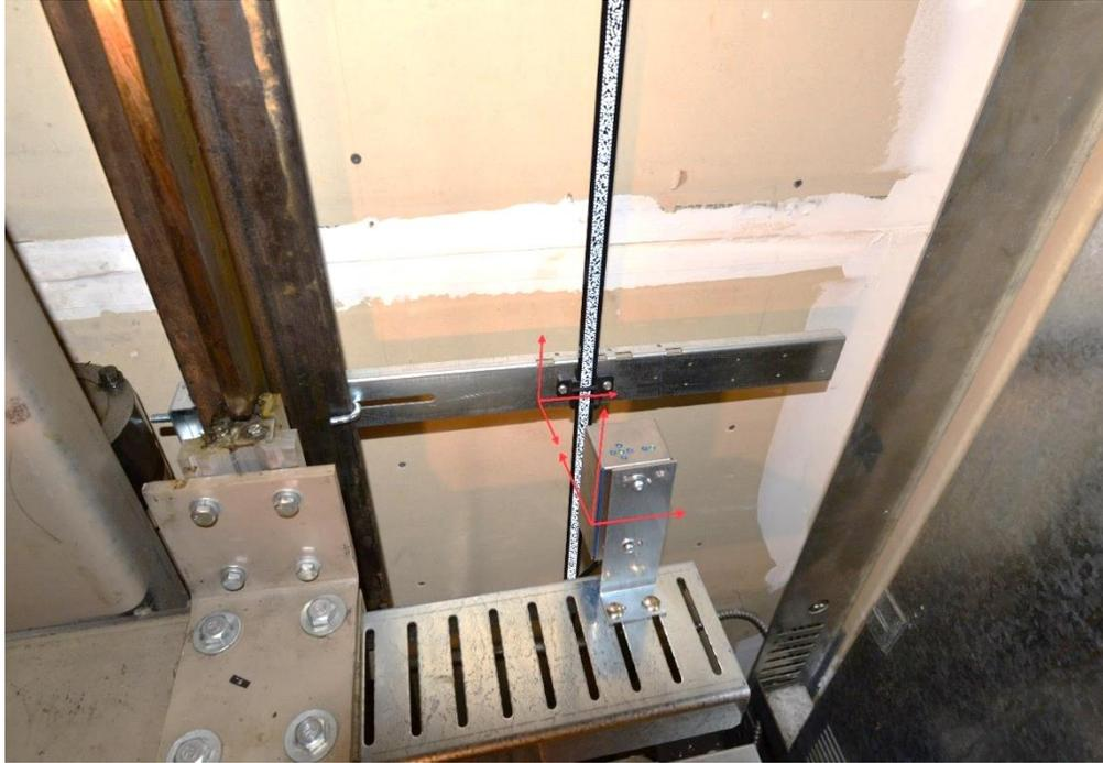
**Figure 2-17: APS Camera Orientation**
