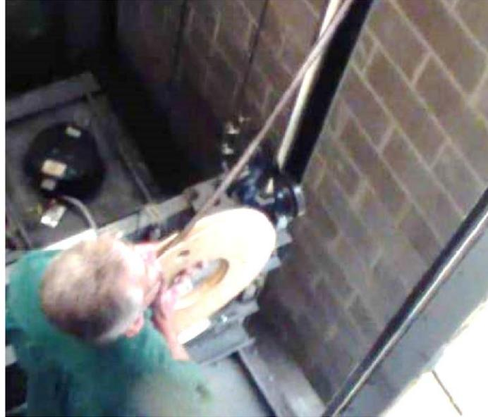
**Figure 2-4: Unroll the Encoded Tape**
