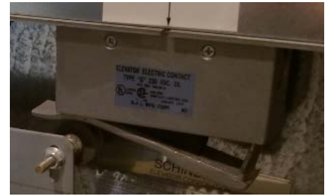
Figure 2: Existing Gate Switch
