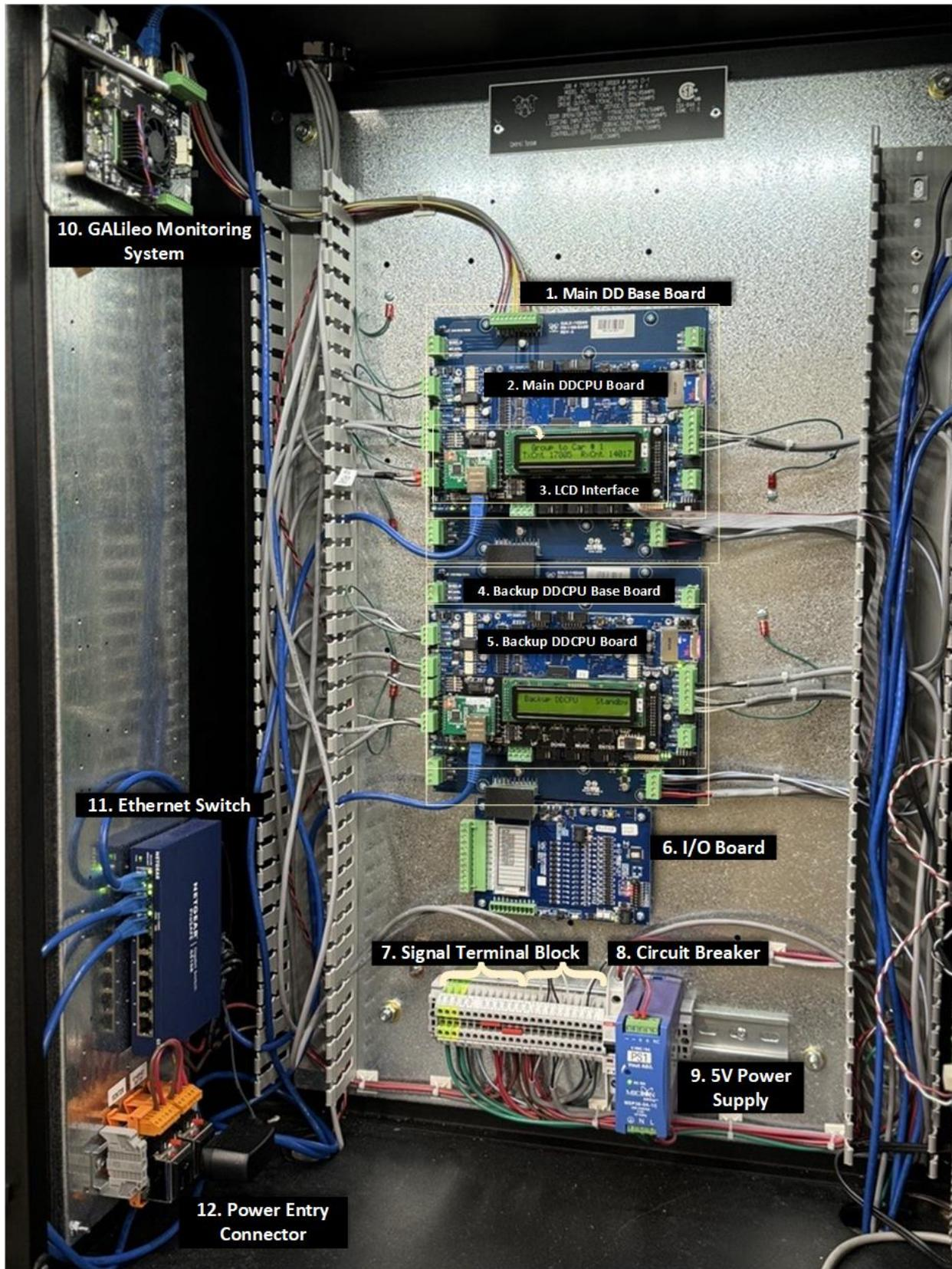
Figure 1-2: Typical Layout of the Controller Top Cabinet
