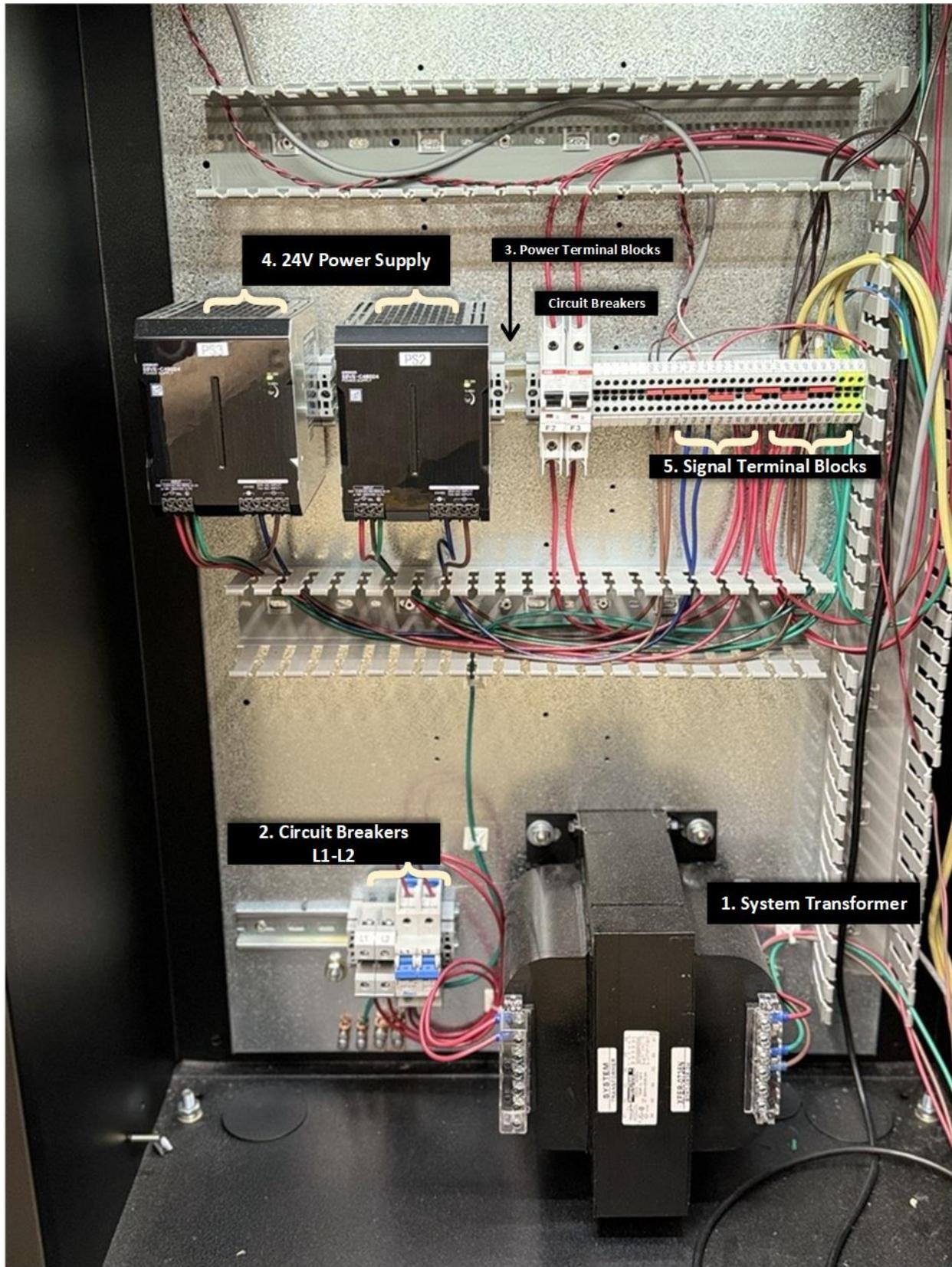
Figure 1-3: Typical Layout of the Controller Bottom Cabinet
